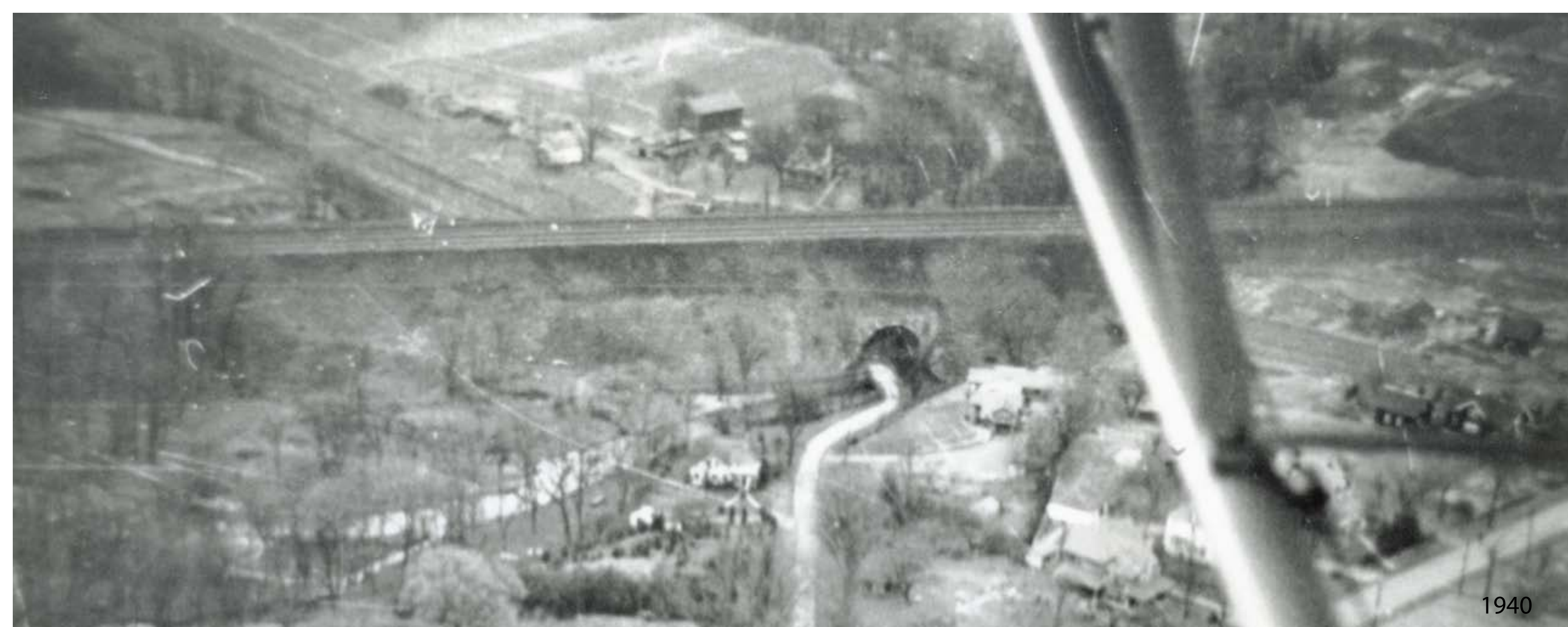
1940 air view of the Great Embankment looking north.
