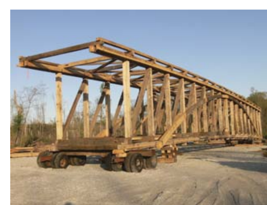
Photo of a "Burr truss" commonly used in the period for both railroads and covered bridges.
