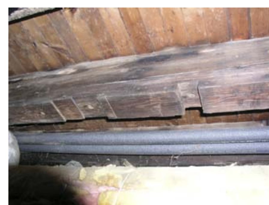
Beam from the trestle re-used as a structural timber in the Corbett house built in 1896. Some of the wooden timbers of the central span were removed to make room for the tunnel when the trestle was buried.
