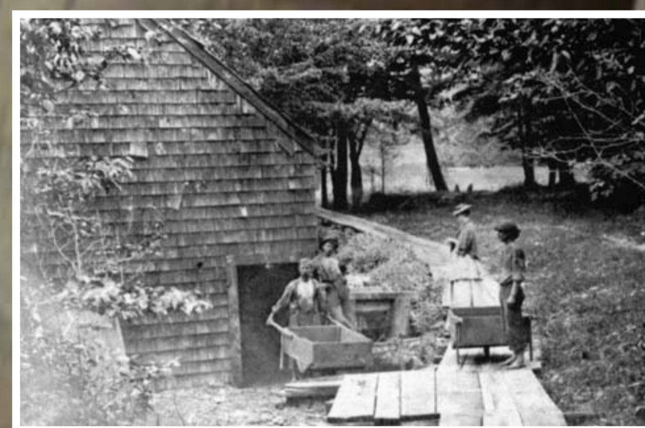
This undated photo of the powder mill in Buckfield Maine shows the wooden walkways that mills used to avoid possible sparks caused by stones on the path.
